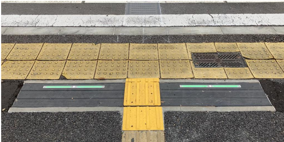
Trough-Type Railroad Crossing Support Device for Visually Impaired Persons
